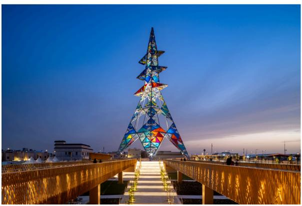
The Arts Tower, 2025 Steel framework with Single-Layer ETFE, featuring 691 colored panels Height: 83.5 meters Base: 33 meters × 33 meters square footprint
